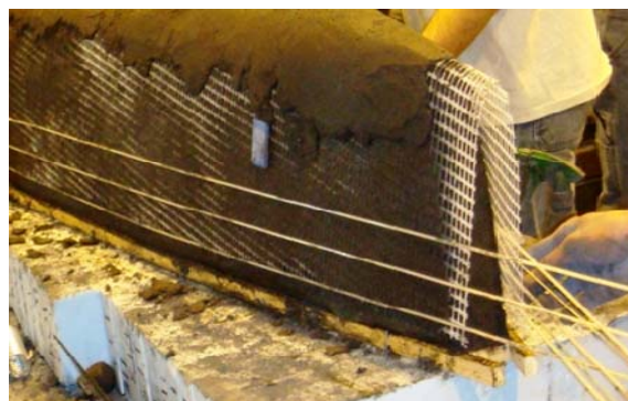
Figure 5 Post-tensioning system installation.
