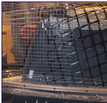
Figure 7: Steel Mesh at Ends.
