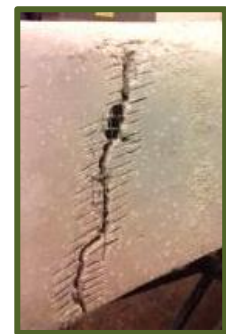
Figure 7: Exposed Reinforcement.
