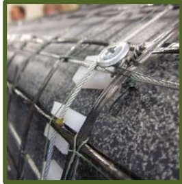
Figure 6: Grade Screw for Depth Control and Tendon
